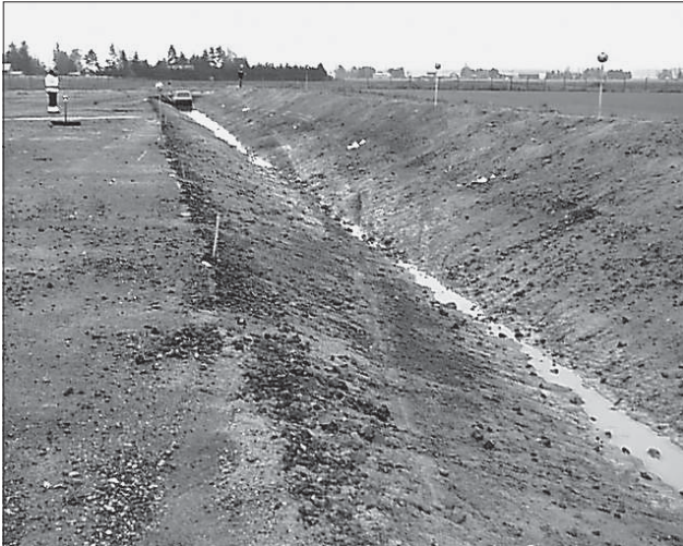
Figure 32. With the more moderate steering manoeuvre the vehicle remained in the ditch but the run was stabile.
