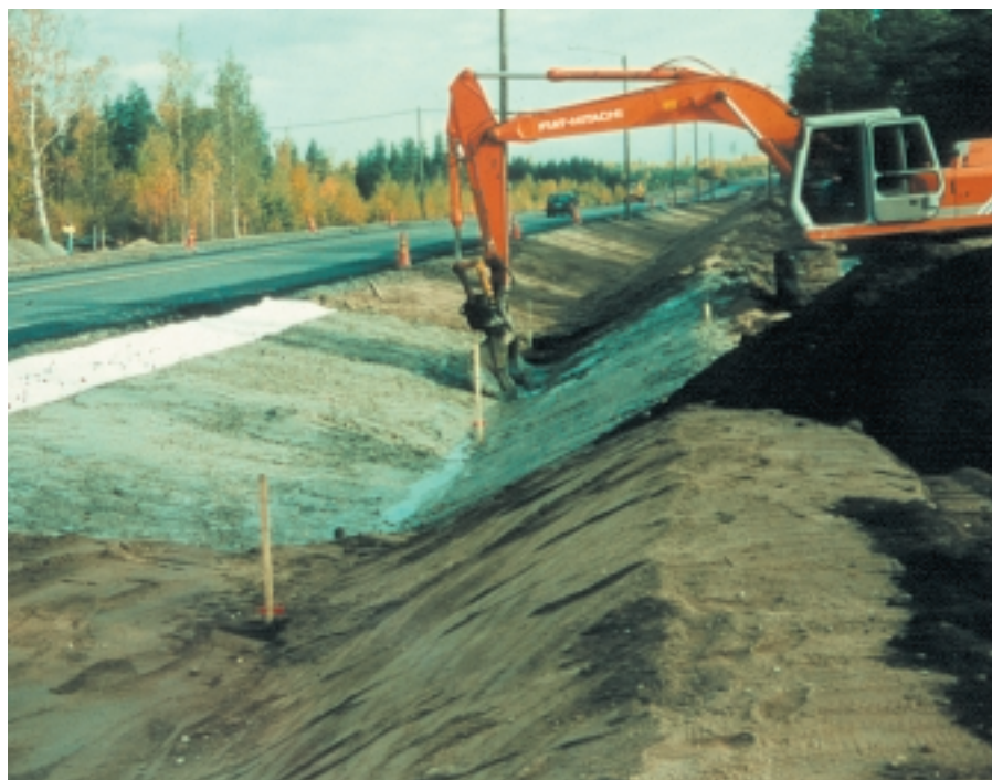
Figure 2. Construction of the Utti glacial clay test target area in August, 1996. The compaction of the clay material was done with an excavator scoop. The groundwater protection of the edge of the pavement (inner slope of the road) was made by using the GCL visible in the picture (light-coloured strip).
