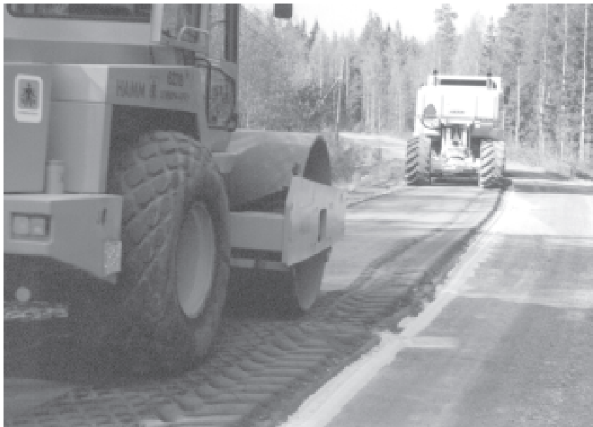
Structure 5. Slag-ash stabilization (the old structure is stabilized to a depth of 200 mm using a mixture of powdered slag and light ashes; this is covered with a 100 mm layer of crushed gravel).
