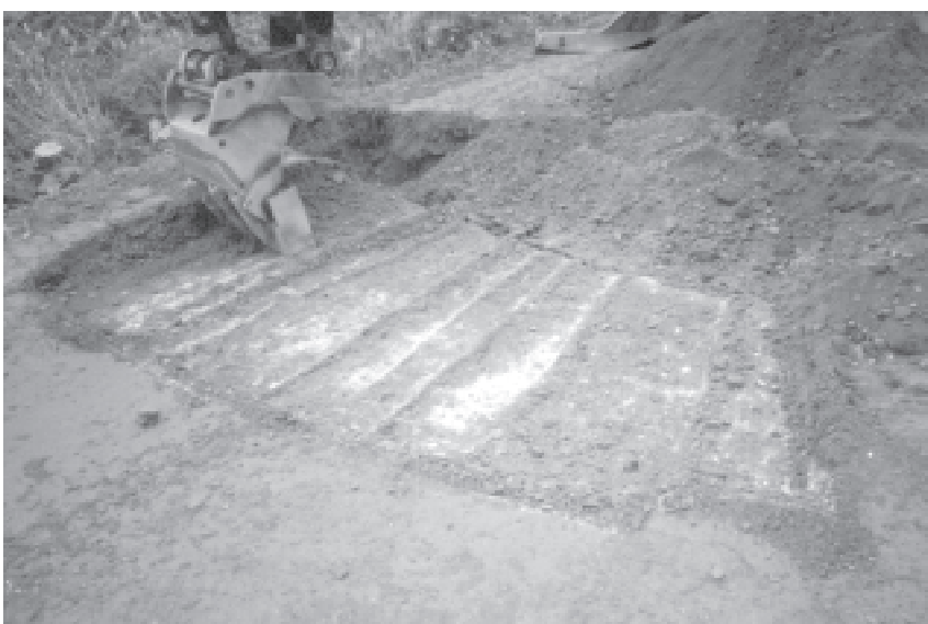
Structure 3. Blast-furnace sand stabilization (the old structure is stabilized to a depth of 200 mm using blast-furnace sand; this is covered with a 100 mm layer of crushed gravel).
