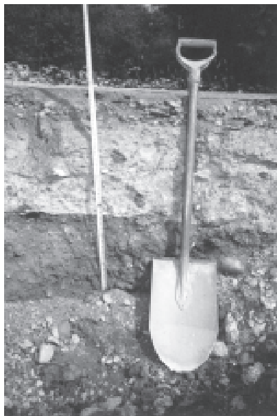
Structure 4. Gypsum-lime stabilization (the old structure is stabilized to a depth of 200 mm using a mixture of gypsum and lime; this is covered with a 100 mm layer of crushed gravel).
