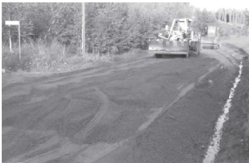
Structure 1. Fibrous ash structure (a 200 mm layer of fibrous ashes covered with a 100 mm layer of crushed gravel).
