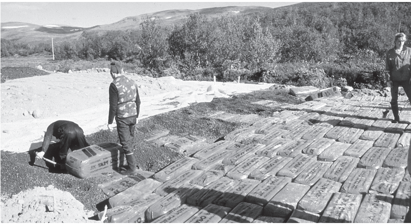
Figure 2. Sacked peat is used as thermal insulation in a road structure.
