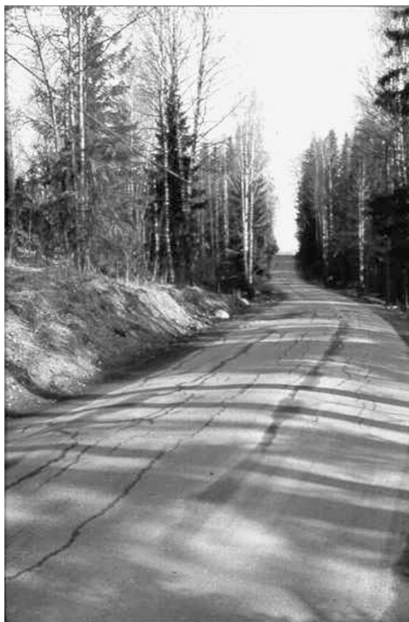
Figure 2. By means of PMS deteriorated road sections can be discovered and compared with each other.
