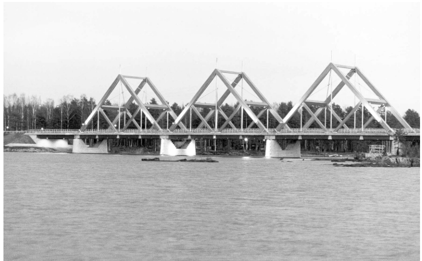
Vihantasalmi bridge, Mäntyharju, Finland. Total length of the bridge 182 metres.
