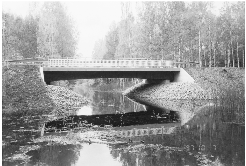
Tirva bridge, Valkeala, Finland. A timber-concrete composite beam bridge.
