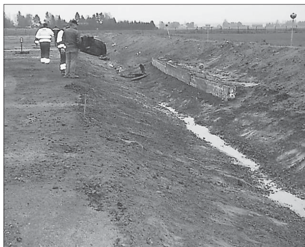
Figure 38. The vehicle did not left skid marks to the frontslope.
