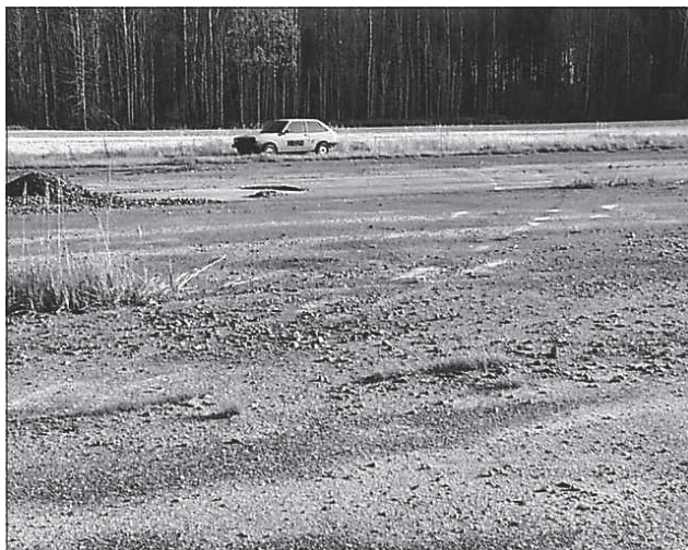
Figure 25. The right tyres hardly crossed the edge of the ditch before the vehicle turned out from the ditch.
