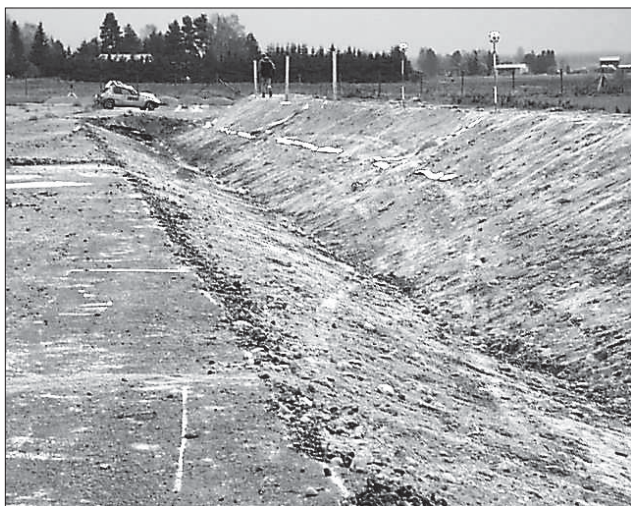
Figure 14. The vehicle turned back to the "road" from backslope. The right side tyres crossed the cross slope and the vehicle rolled over.
