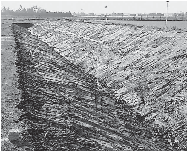
Figure 10. The vehicle path in the ditch
