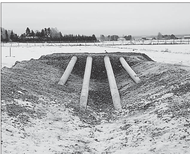
Figure 2. Crash attenuator for cross slope made by wooden columns.
