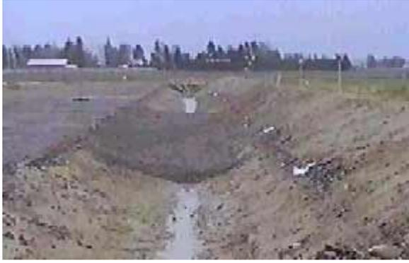
FIGURE 4: U Shaped Ditch (Loose Gravel Bottom)
